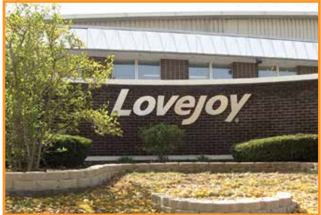
Lovejoy, LLC World Headquarters in Downers Grove, Illinois USA
