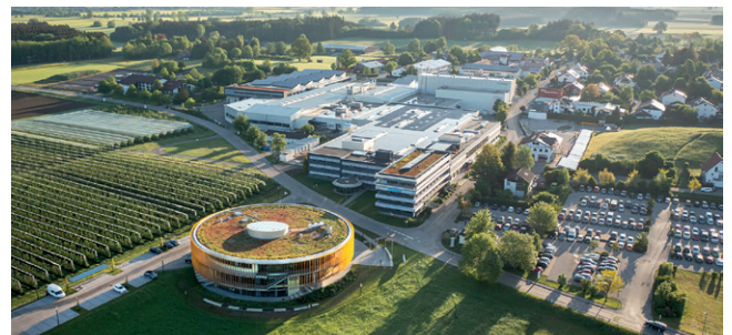
mayr ® headquarters in Mauerstetten
