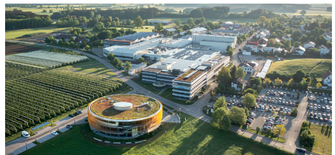
mayr ® headquarters in Mauerstetten
