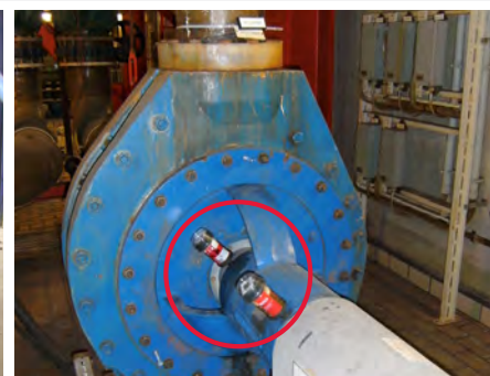
Drive shaft lubrication on a pump
