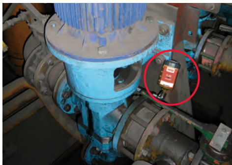
Fuel pump lubrication in the refinery process
