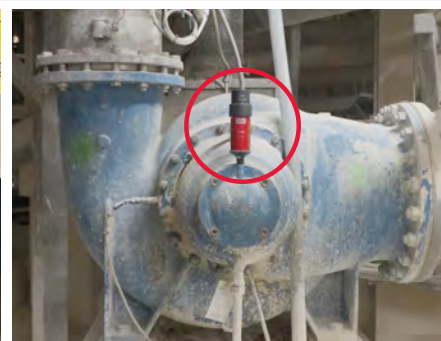
Bearing lubrication on a pump
